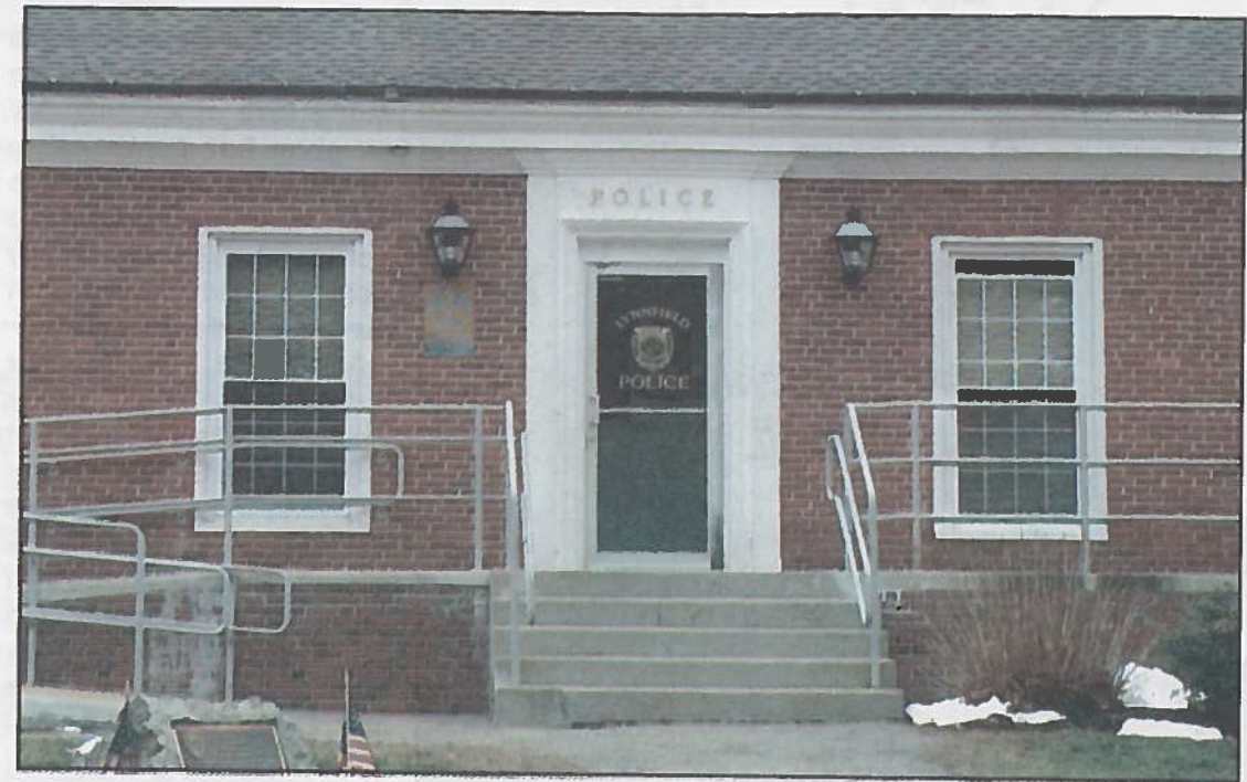
Lynnfield Police Headquarters has a number of space and infrastructure issues that have only become worse in recent years.
